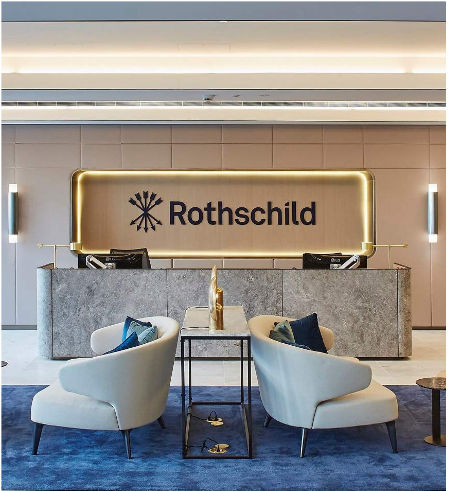
Feature Recess in Reception Wall - Timber Veneer with Metal Surround
